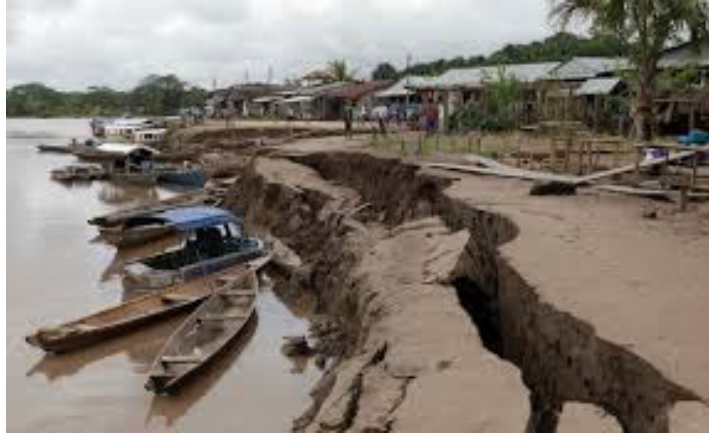
The banks of the Huallaga River are cracked after an earthquake in Puerto Santa Gema, on the outskirts of Yurimaguas, Peru, Sunday, May 26, 2019.
